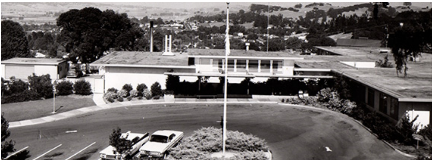
New 50-bed Hillcrest Hospital opened 1957 by the Petaluma Hospital District. Courtesy of Petaluma Health Care District.
